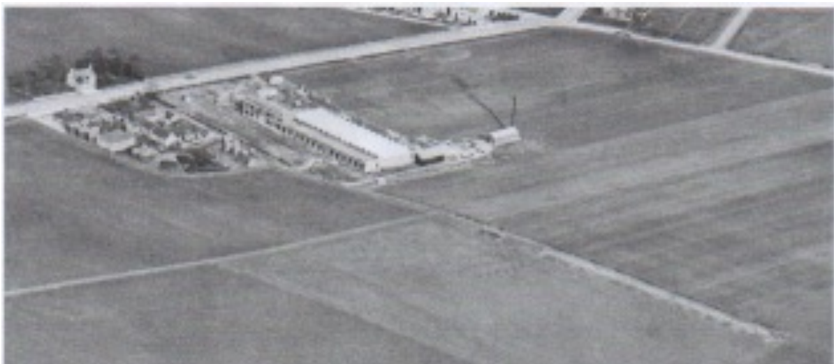
Aerial photo of King's Buildings in early 1921
